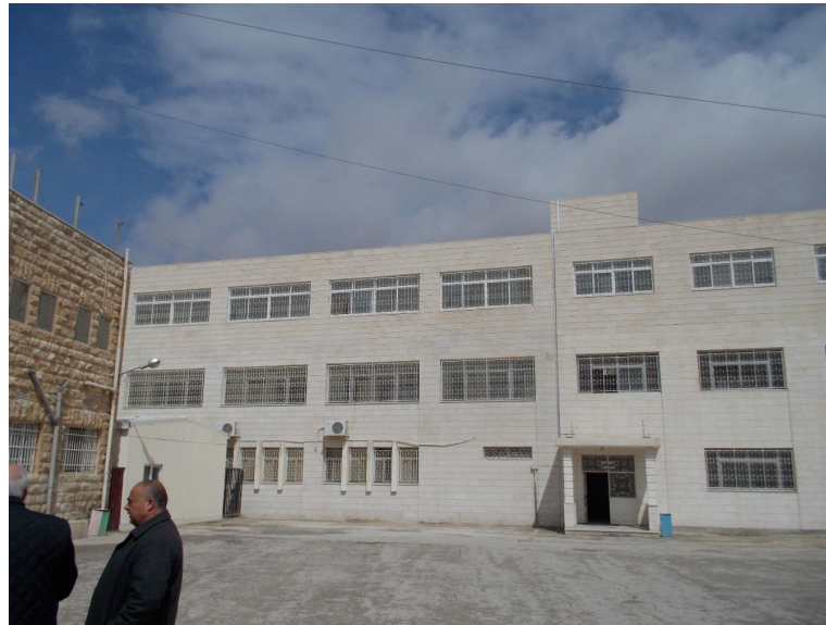
Mafraq Jordan School 2015 Expansion Project
